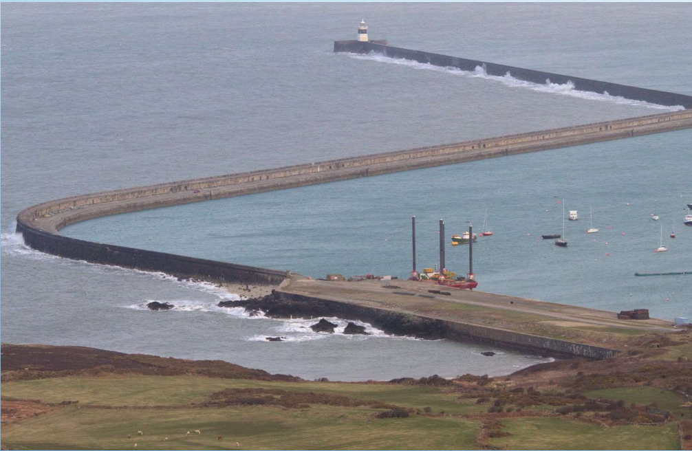
Holyhead Breakwater UK, L=2.74km
