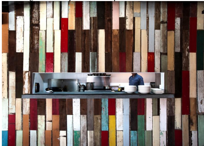
Figure 15: Recycled wooden planks on kitchen wall
