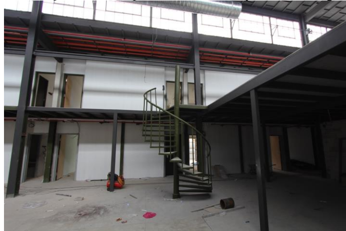
Figure 7: Reused spiral fire escape staircase in lobby from the original structure
