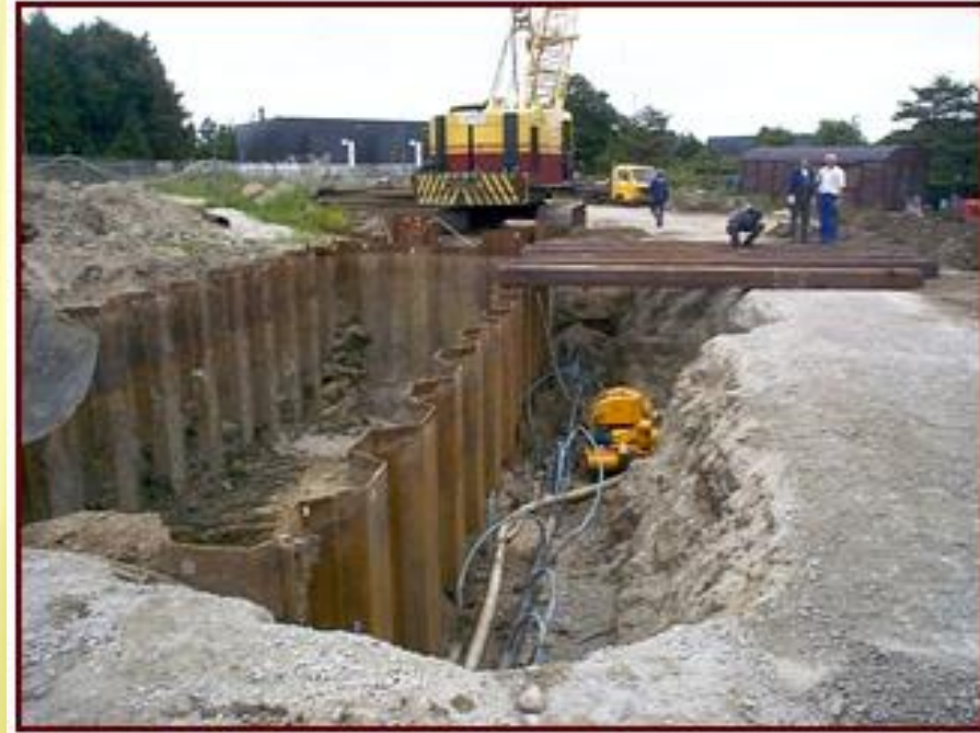
PRB before removing sheet pile
